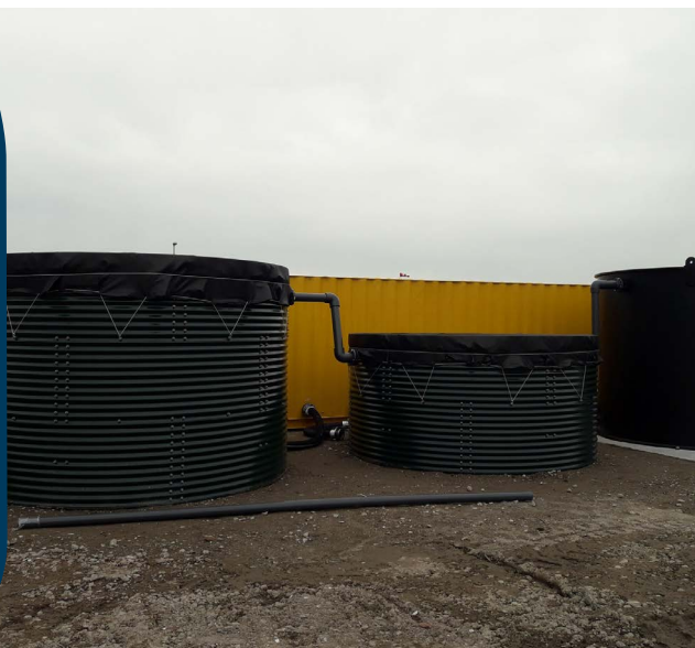
Two activated carbon filters for removal of PFAS at drinking water site
